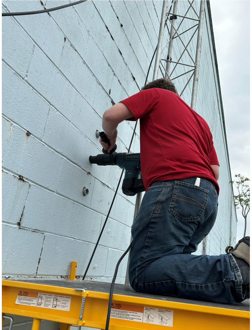
Dan KD9KFJ drills new access holes for the repeater's coax
